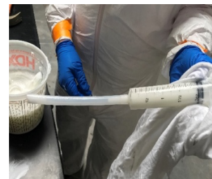
Figure 2 Mixing saturating epoxy (left) and putty (center) for anchor saturation and installation. A 60cc syringe, or similar is used to fill anchor holes 1/2 to 2/3 full (right).
