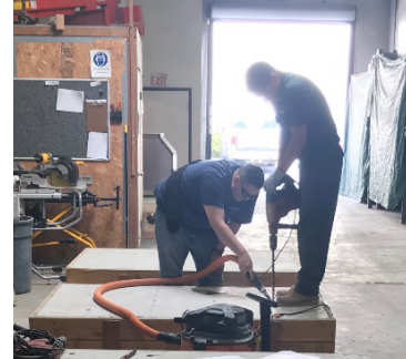
Figure 1 Typical drill and steel bristle brush for cleaning (left and center). Drilling with vacuum assistant (right).
